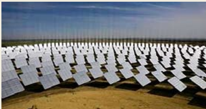
Solar furnace at Sanlucar La Mayor, near Seville, uses an alternative technique with mirrors angled to heat a chamber on top of a tower
